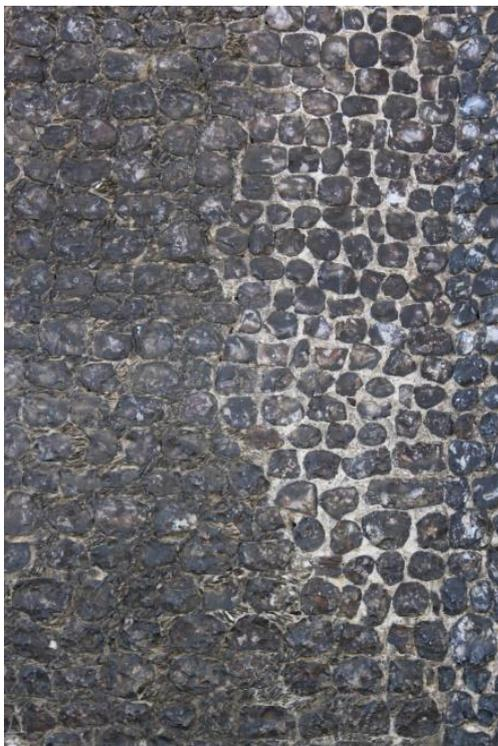
Fig. 4 shows a small area of wall which is located on the same façade as seen in Fig. 3. This illustrates the black effect of the flints in combination with matching gallets. The recent repair may be a temporary intervention to protect the flints from weathering and possible detachment but it helps to illustrate the damaging effect of omitting a significant element of the fabric. The ambience of the area is affected by the sharp contrast.
